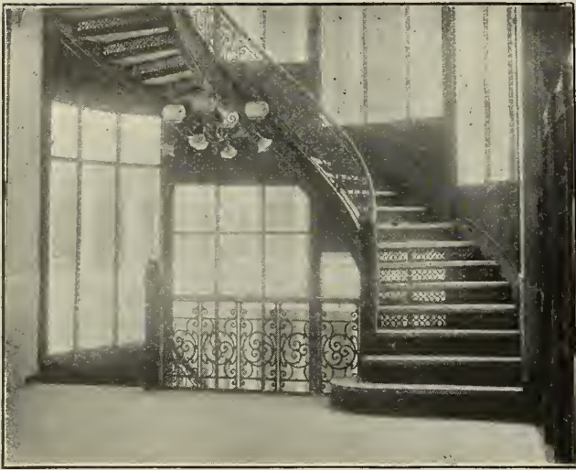
A.—ORIEL STAIRCASE, MILLS BUILDING, SAN FRANCISCO. Wrought Iron Rail, Cast Iron Stringers and Risers.
